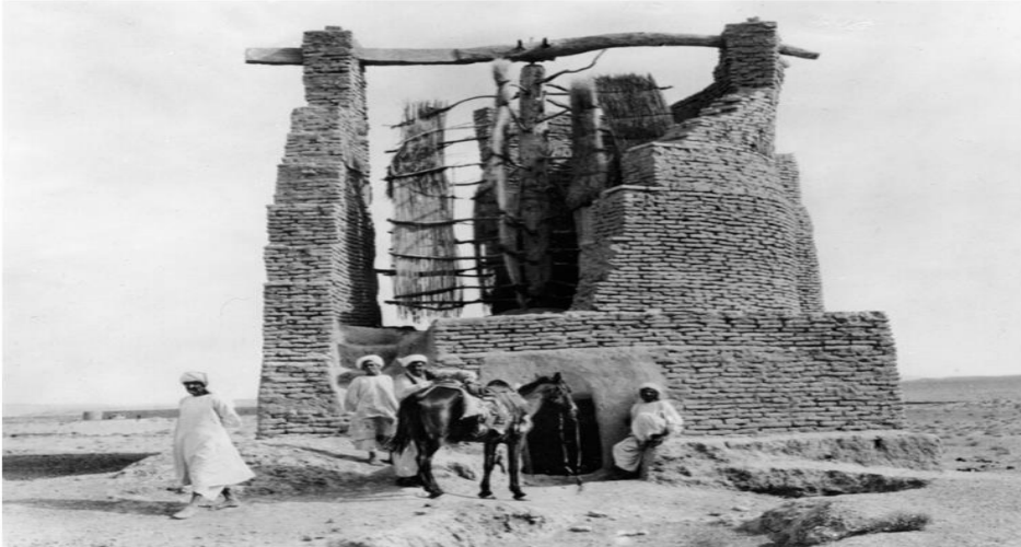
Vertical-axis windmill for milling grain, Afghanistan
