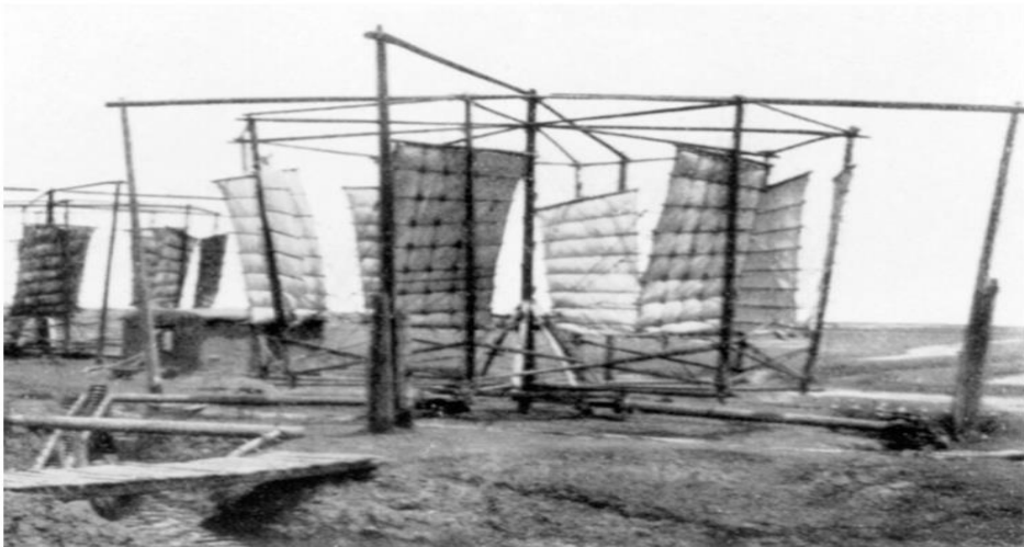
Ancient Chinese windwheel for pumping water
