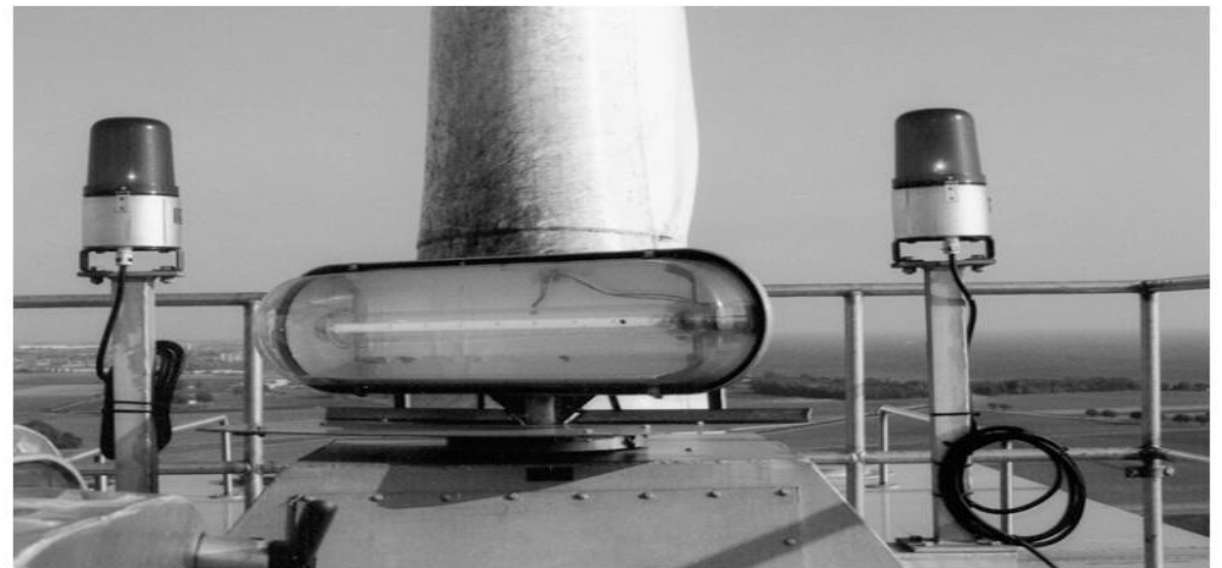
Safety lights (night-time markers) on the WTS-3 in Maglarp with omnidirectional beacons or also rotating flashing lights (Sweden)
