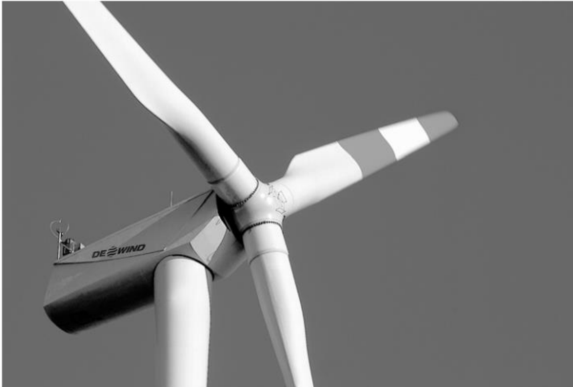
Daytime markings on the rotor blades of a Dewind D-6 turbine
