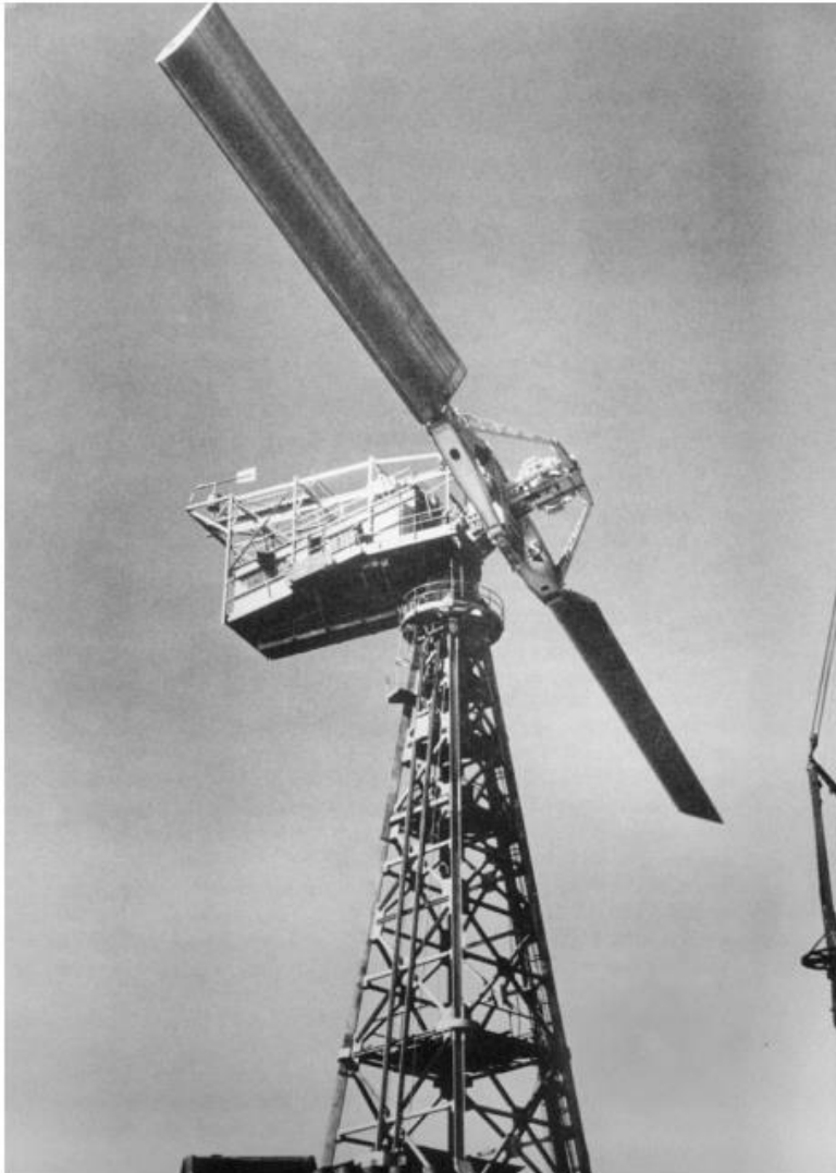
Smith-Putnam wind turbine, in Vermont, USA (rotor diameter 53.3 m, rated power 1250 kW), 1941
