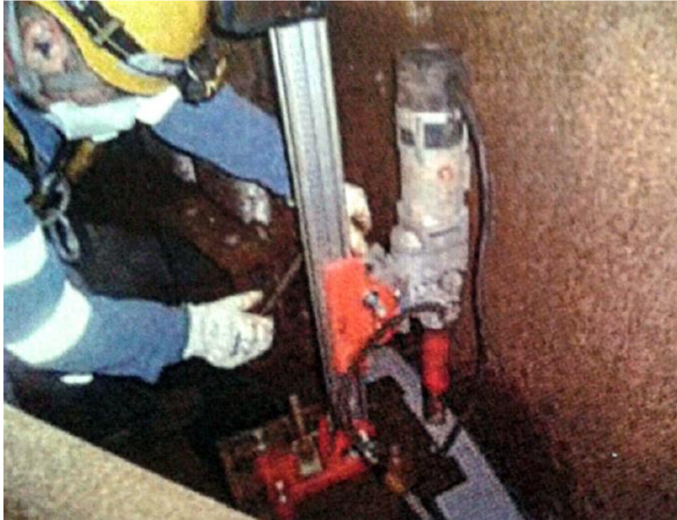
Core drilling
