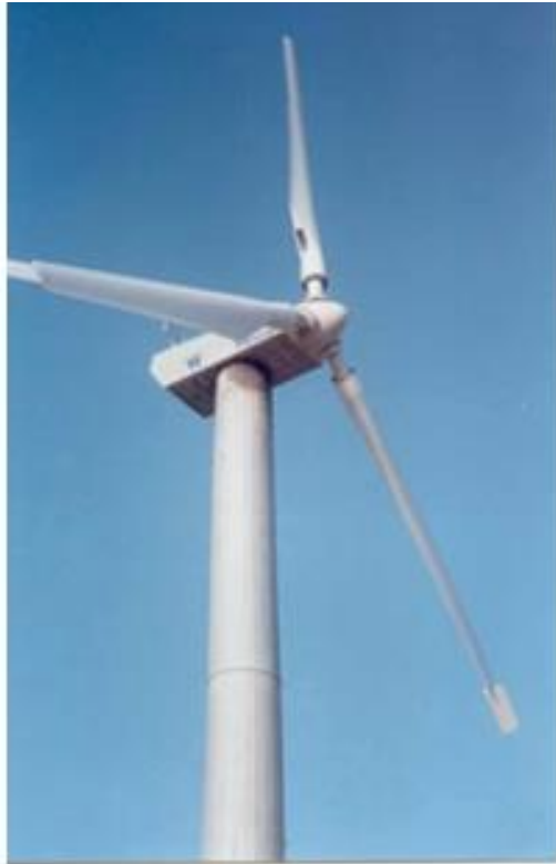
1997: The 1st Greek 9.3m blades during installation on 110kW W/T CRES wind park at Lavrio
