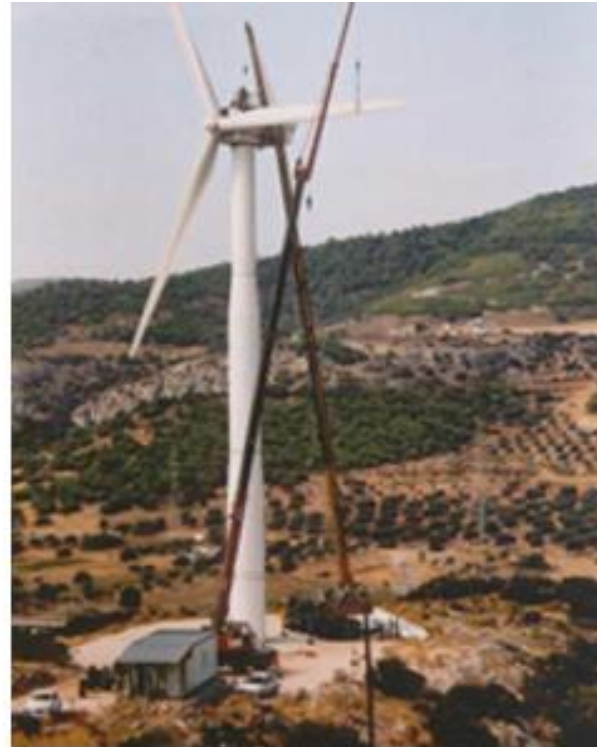
2001: Greek 19m blades installation on Greek 600kW wind turbine CRES wind park at Lavrio
