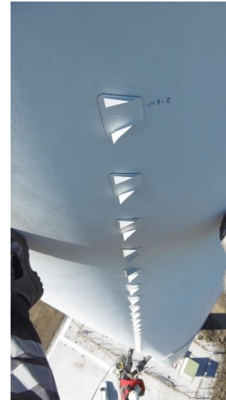
3M Vortex Generators installation at Turkey on 2.5MW (2017), Compblades is VG's certified installer
