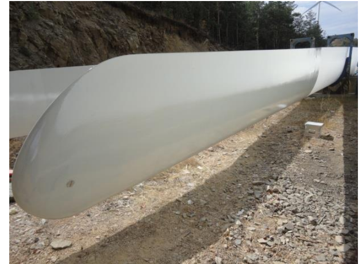
5m skin replacement in 40m blade without moving or turning the blade
